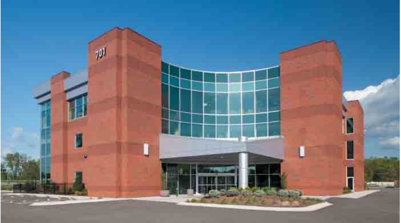
CLEAR CHOICE To take advantage of greenery surrounding the building site, and to make the structure come alive when viewed from outside, building corners are essentially glass.
